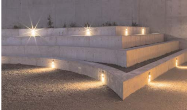
Square Steps Star™ fixtures illuminate the amphitheater. Photo Credit: Nic Lehoux
