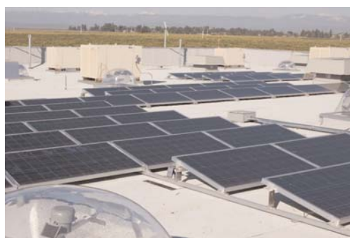
Solar Panel installation began in 2007
