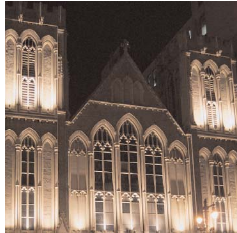
More than a dozen Sierra Series™ fixtures now adorn the facade of the Chambers Wylie Church in Philadelphia. Photo Credit: The Lighting Practice
